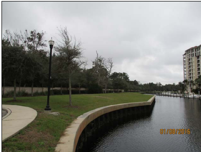
Project site with views of the marina basin.
